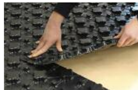
Installation of System Plate
